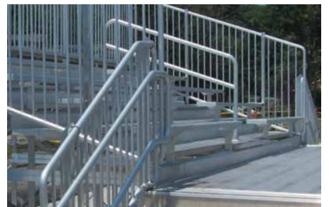
VERTICAL PICKET GUARDRAIL
