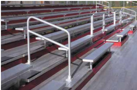
AISLE WITH HANDRAIL
