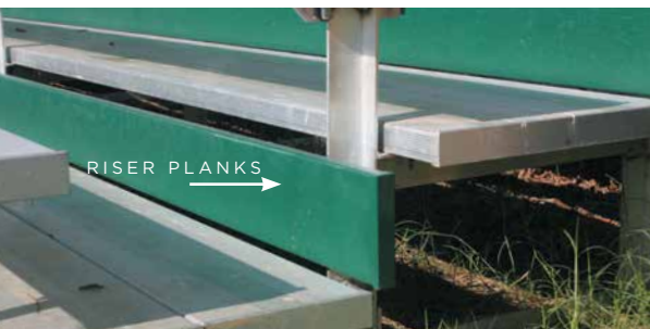
RISER PLANKS ON ALL ROWS
