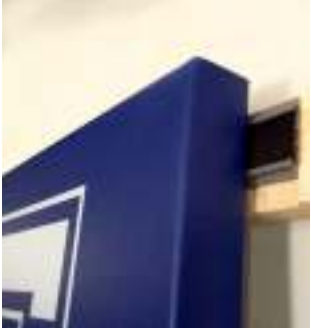
Wood Backed Velcro® Track Mounting System
