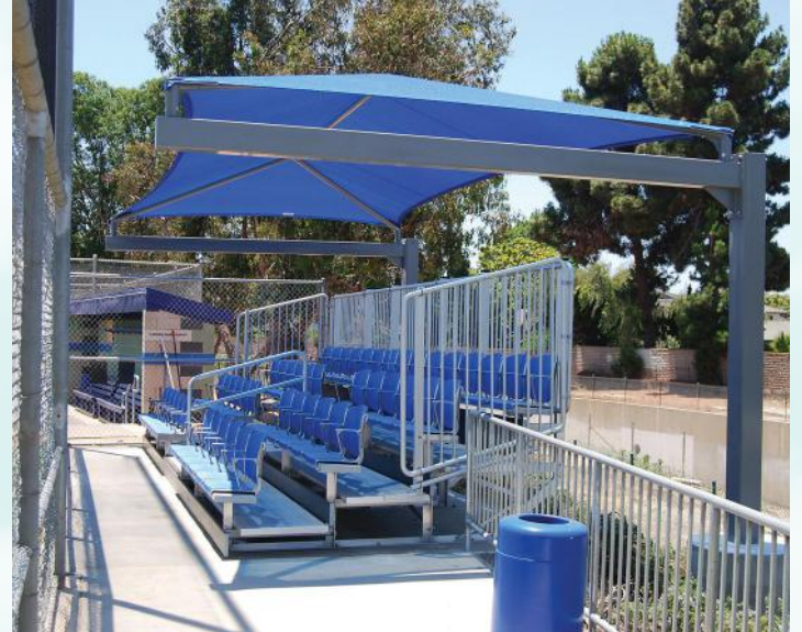
WINDWARD HIGH SCHOOL, LOS ANGELES, CA
